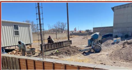
Construction of the warehouse is progressing.
