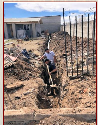
A brand-new sewer line at the base.
